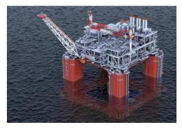
The development involves a wet tree subsea system connected to an infield floating production unit (FPU), which will be linked to a floating storage and offloading (FSO) unit, ensuring efficient extraction and processing of the resources.
